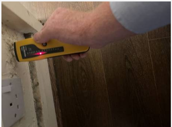
Hallway (Basement) — photograph 16
