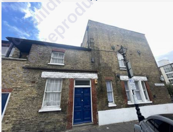
External Elevations — photograph 4
