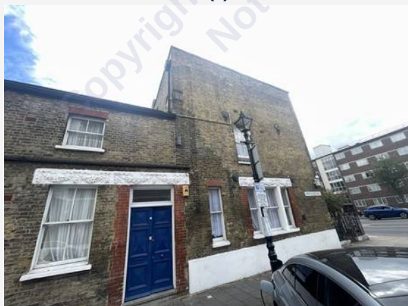
External Elevations — photograph 5
