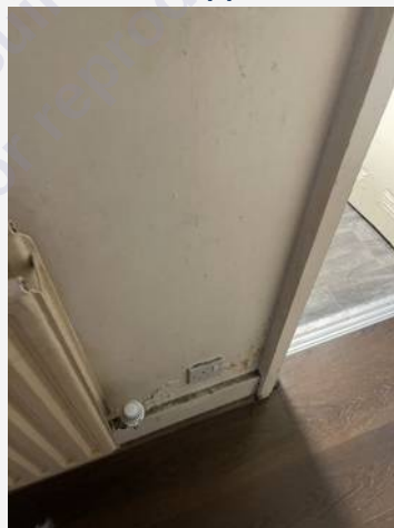
Hallway (Basement) — photograph 4
