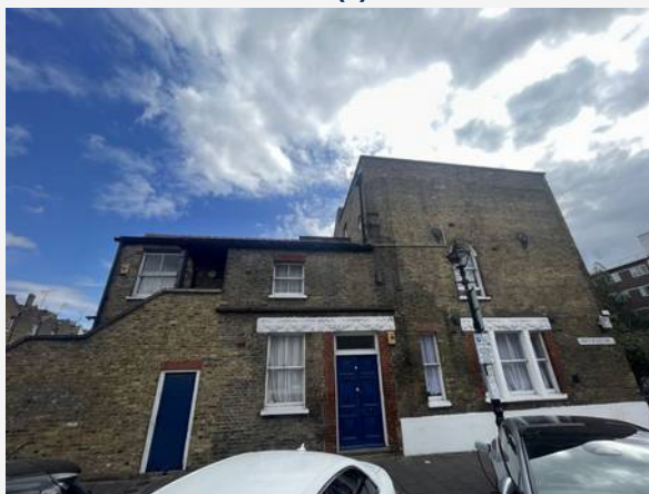
External Elevations — photograph 6
