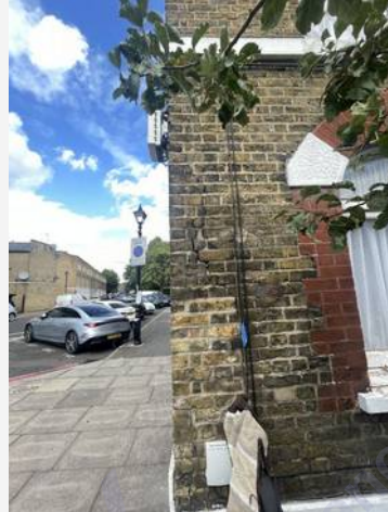
External Elevations — photograph 8
