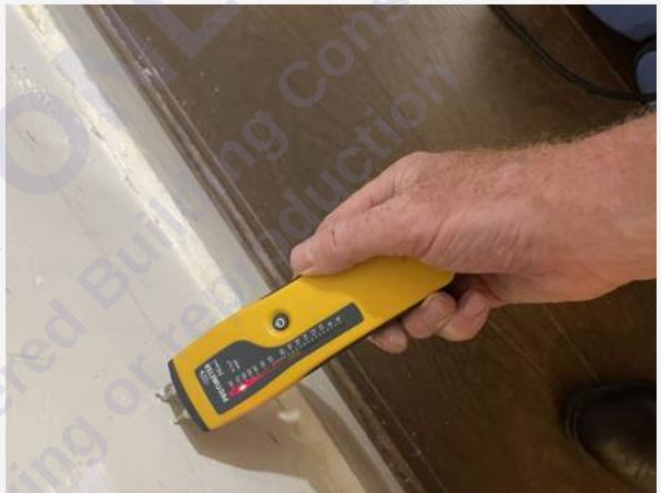
Hallway (Basement) — photograph 14
