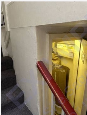
Cellar (Basement Store) — photograph 3
