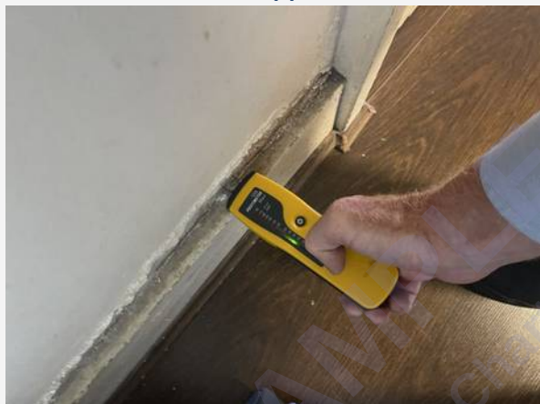
Hallway (Basement) — photograph 7
