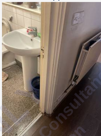
Hallway (Basement) — photograph 2
