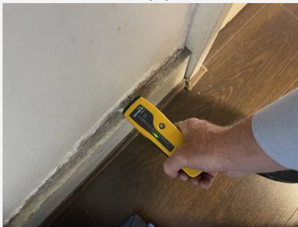
Hallway (Basement) — photograph 10
