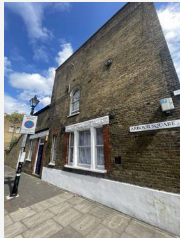
External Elevations — photograph 12
