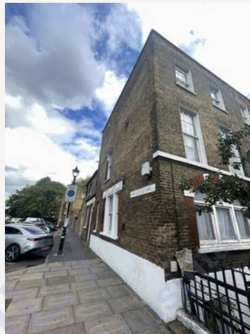
External Elevations — photograph 2
