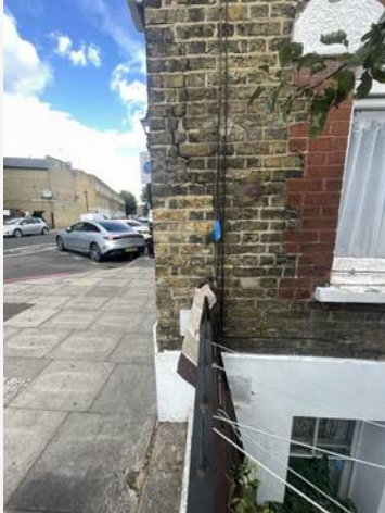
External Elevations — photograph 7
