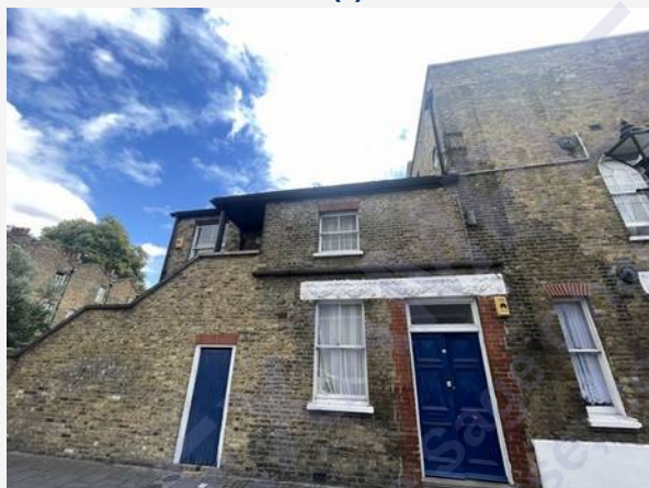
External Elevations — photograph 3
