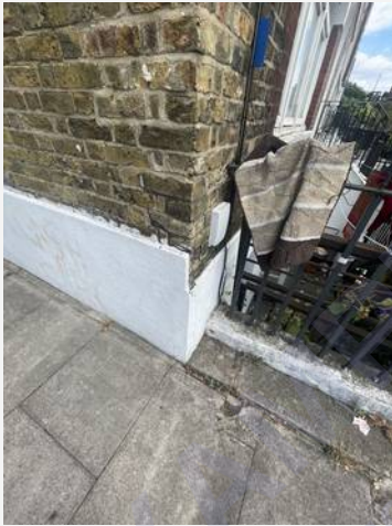
External Elevations — photograph 9
