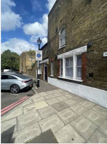
External Elevations — photograph 13
