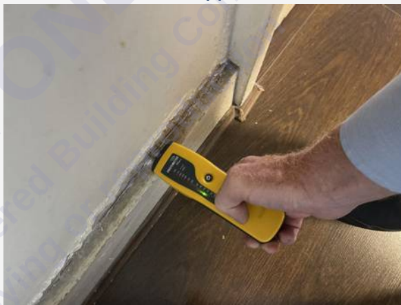
Hallway (Basement) — photograph 8
