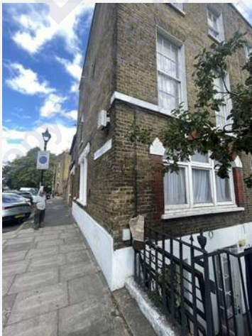
External Elevations — photograph 11
