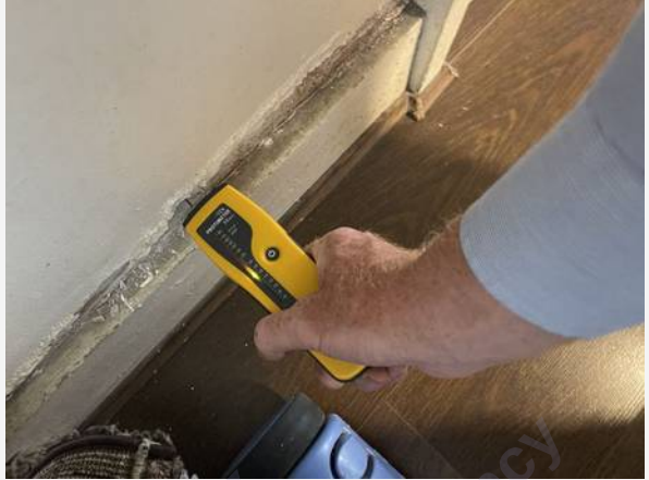
Hallway (Basement) — photograph 12
