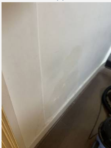
Hallway (Basement) — photograph 5
