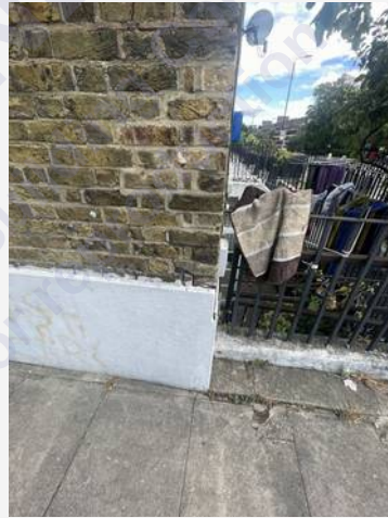
External Elevations — photograph 10
