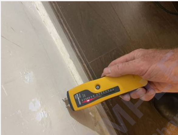
Hallway (Basement) — photograph 13
