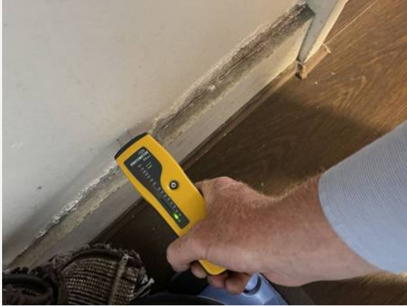
Hallway (Basement) — photograph 11
