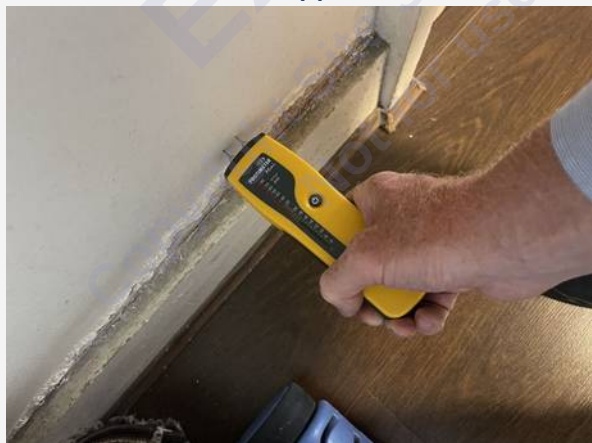
Hallway (Basement) — photograph 9
