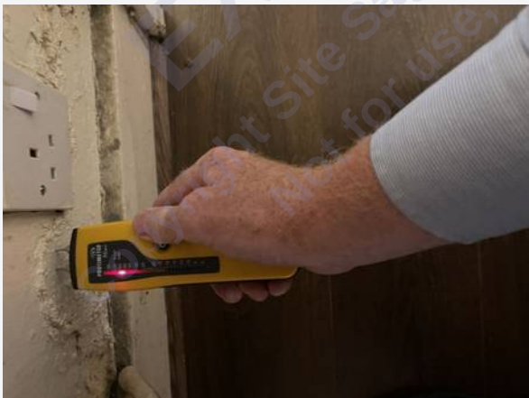
Hallway (Basement) — photograph 15
