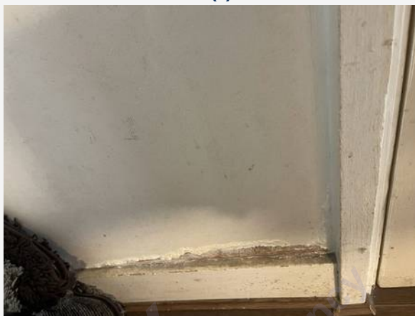
Hallway (Basement) — photograph 6
