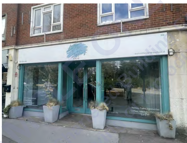
The front elevation and shop front to Sample Road
