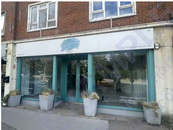
Plate A3 The shop front. Flat fascia carrying applied vinyl graphics, glazed screen and entrance doors in painted frames.
