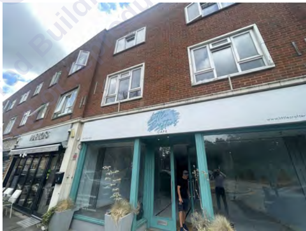
Plate A4 The entrance doors standing open. Applied vinyl lettering to the glazing on both sides of the entrance.
