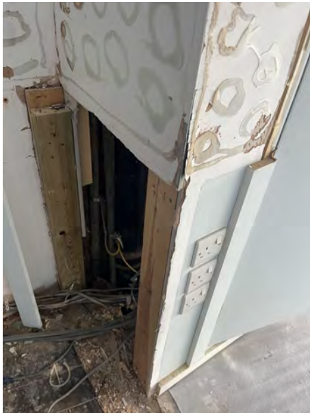
Plate H5 The boxing in seen from the rear room, cut away on a diagonal and left unfinished, with services exposed within.
