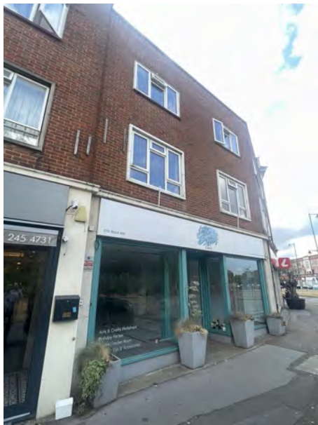
Plate A1 Oblique view of the parade from the north-west. Three storeys of facing brickwork over the ground floor shop units.
